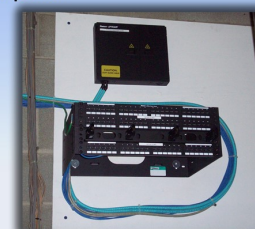
Wall mount patch panel and fiber optic panel
